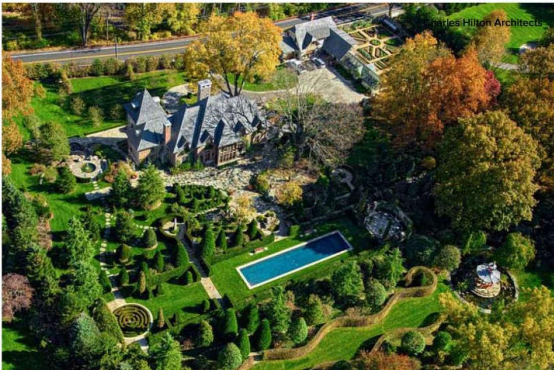
Despite the estate's historic look and feel, Hilton says that "we incorporated lots of modern technologies, including a geothermal cooling and heating system, energy-efficient spray insulation, LED lighting, and energy-efficient technologies for water and electricity."
