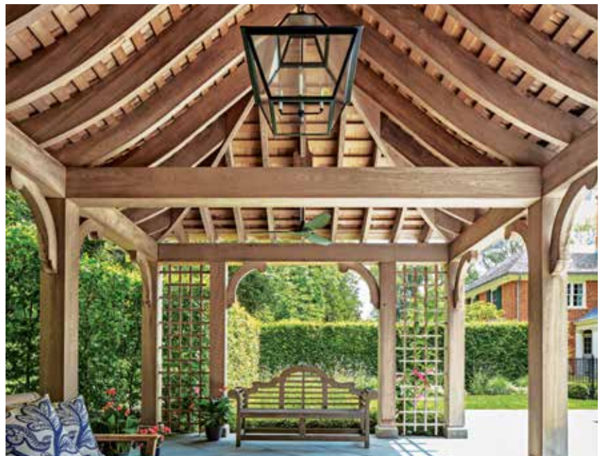
CLOCKWISE FROM ABOVE: A study in geometry, note how the rafters all die cleanly onto the lintels, and the hip rafters form a perfect triangle at the top and bottom. The exposed rafter tails have profiled ends; the decorative detail was created by the team at Charles Hilton Architects. Interior designer Tim Button chose furnishings that are the same color and period as the pergola; the lantern is a custom Paul Ferrante fixture enlarged for scale.
